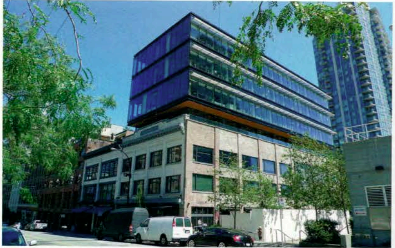
Reliance Properties Ltd. transformed a century-old brick-and-beam building at 564 Beatty into 50,000 square feet of top-class offices | ROB LESHGOLD
